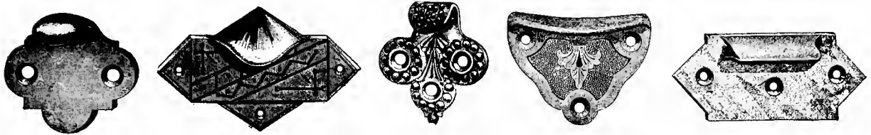
Figs. 4497-4501. WINDOW-SASH LIFTS, CONE AND STRAIGHT TOP.
